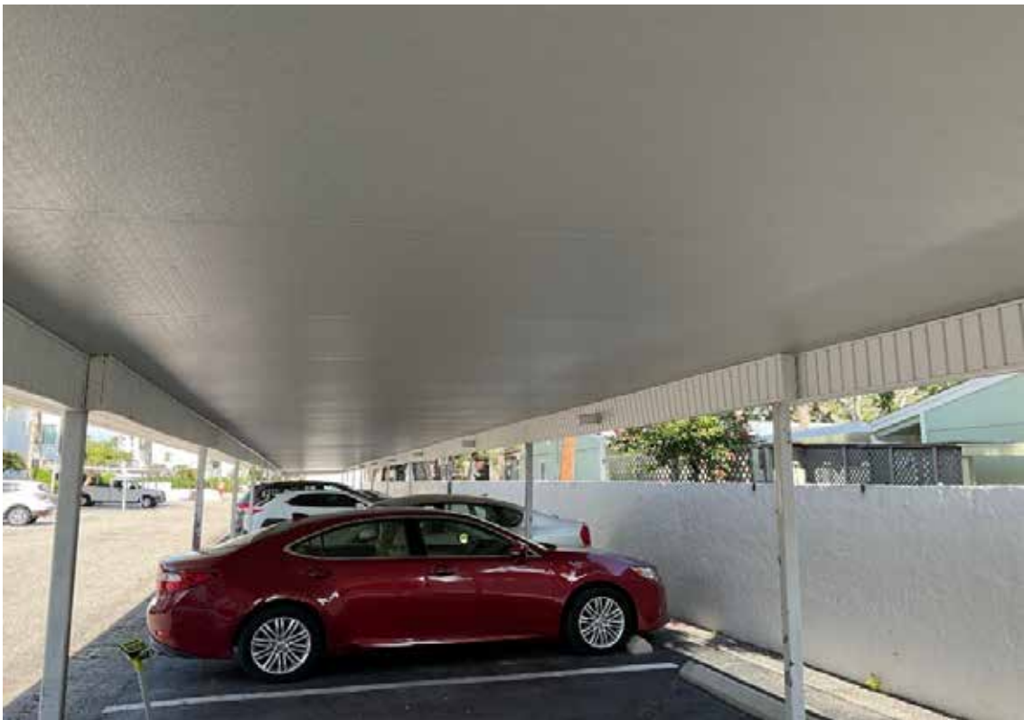
Carport Roof Panels - Typical
