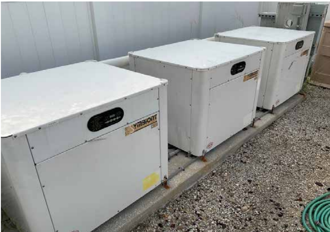
Pool Equipment, Geo-Thermal Heat Pumps
